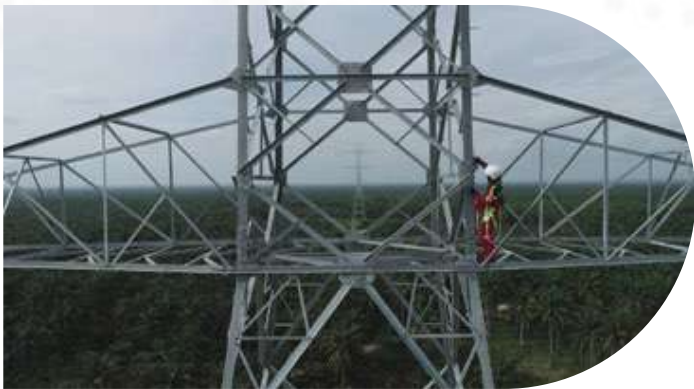
TOWER 500KV JAMBI
