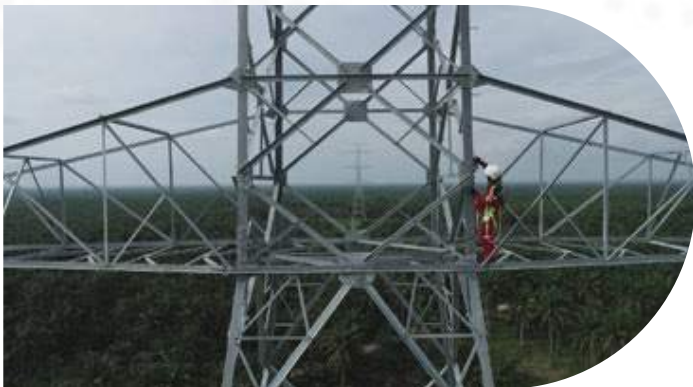
TOWER 500KV JAMBI
